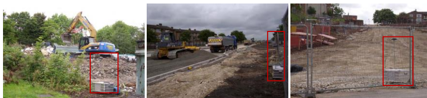
Fig. 1: Positions of dust analyzers. Left: demolition activity. Middle: earthwork. Right: site entrance. Pictures from HSE (HSE, 2011).
